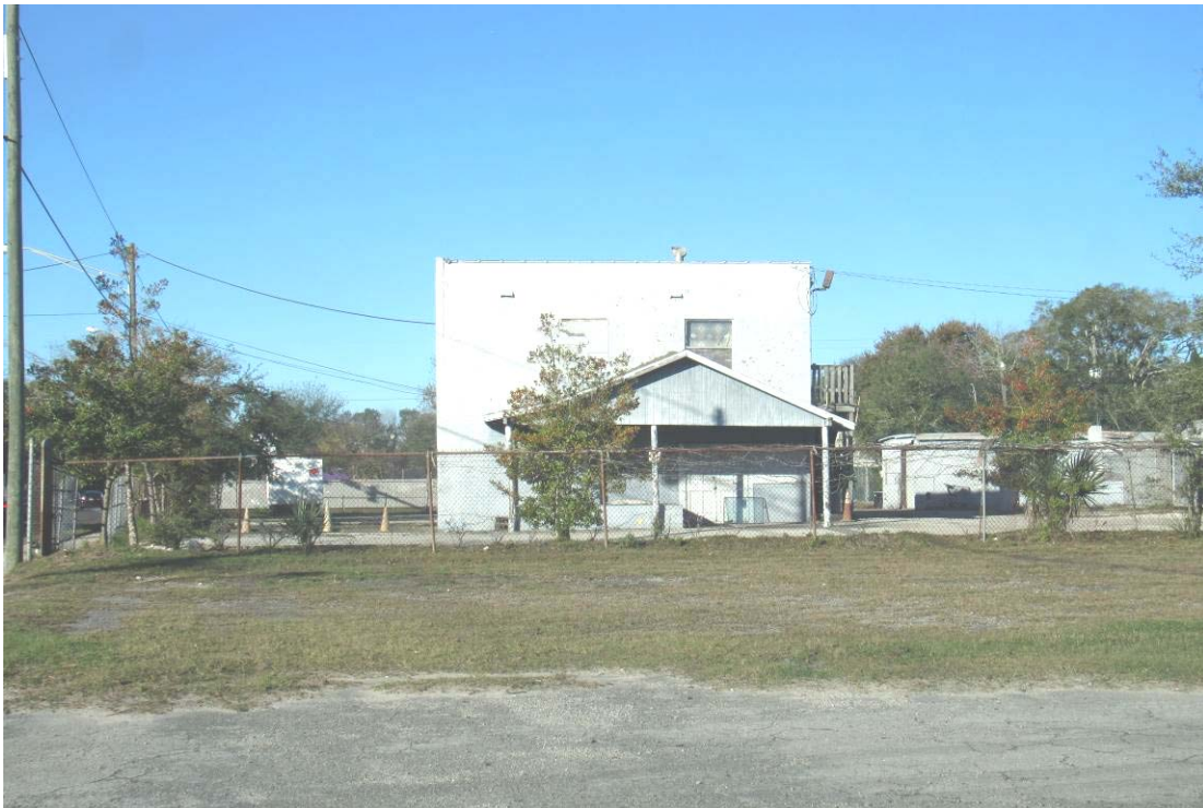
View of existing building on the subject property.
